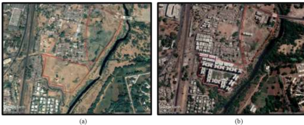
Fig. 4: Construction near Bhimnath bridge (a) 2000 (b) 2019
