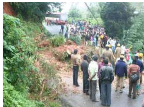
Landslide at Ooty - Coonoor ghat road
