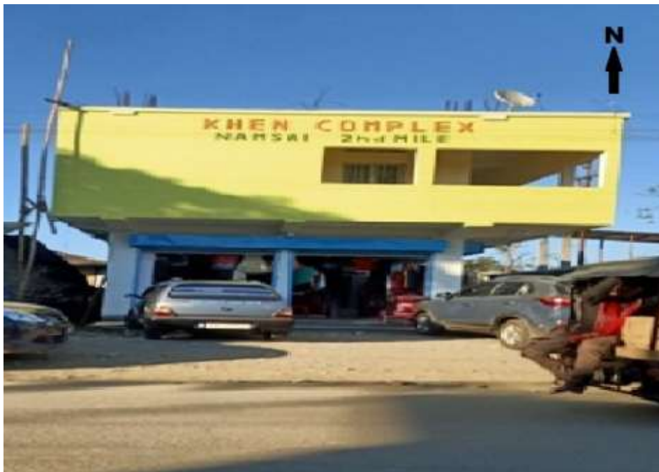
g. Buildings in Namsai town: Designed without following the BIS Code
