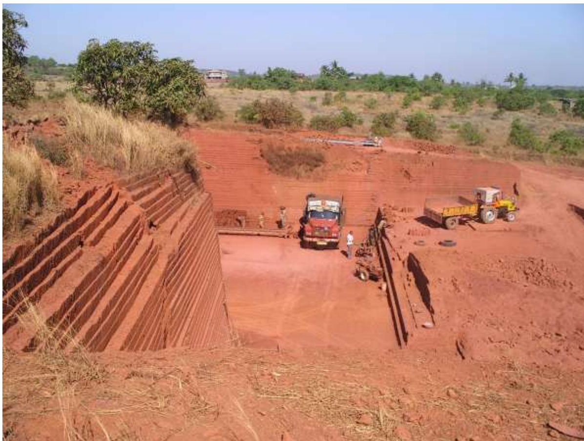
Figure 1: Excavation of lateritic blocks from the lateritic plateau region
